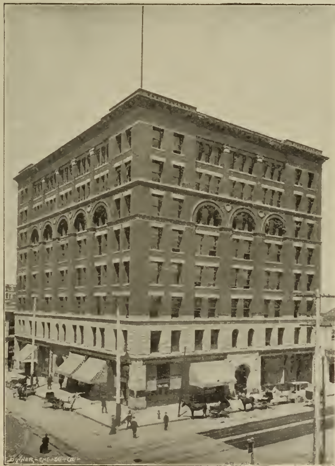
COOPER BUILDING, DENVER, COL. (See ORNAMENTAL IRON, November, 1894.)
